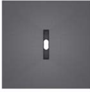
Fundo Riofino square, central drain
